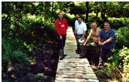
Committee members hard at work laying wooden pallets at Tyn-y-Cerrig
